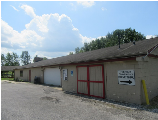
Office building front overview
