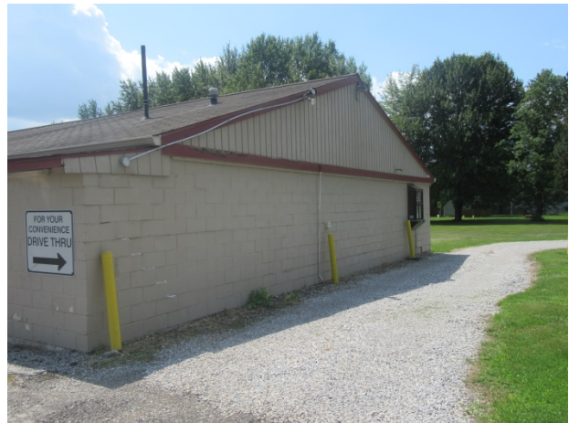
Office building side overview
