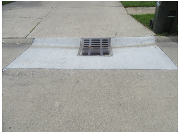
Catch basin replacement at Horseshoe Drive
