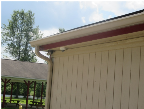
Gutter and downspout assembly
