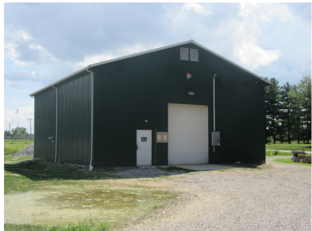
Sewage building side and rear overview
