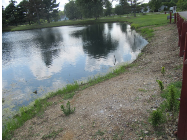
Pond shoreline erosion
