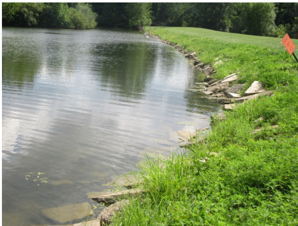
Lake shoreline concrete rip rap
