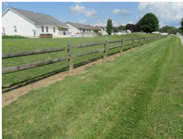
Wood split rail fence; we note organic growth and leaning sections
