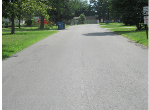
Phase 3 pavement, Hickory Run
