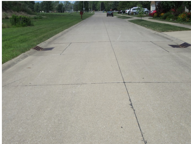
Concrete street, East Lake Drive
