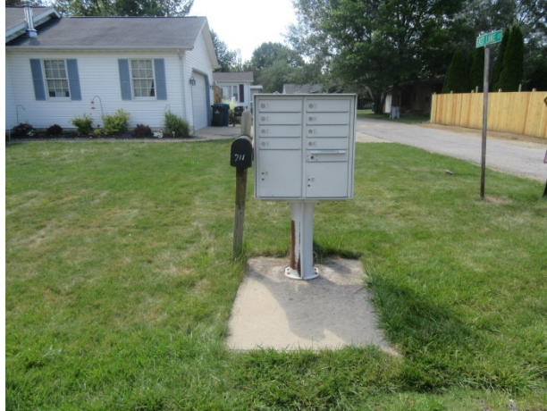
Mailbox station; we note finish deterioration
