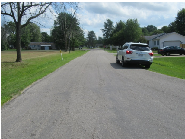
Phase 2 pavement, East Lake Drive; we note cracks
